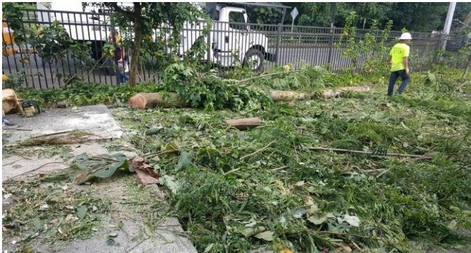
Riverside Apartments - Puueo Street view after tree cutting by Backyard Monkey.
